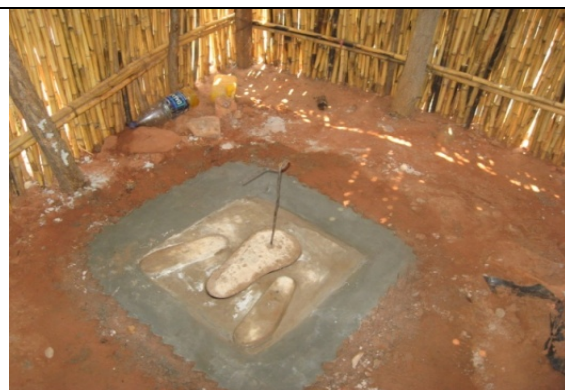
Pit latrine with slab (washable)
