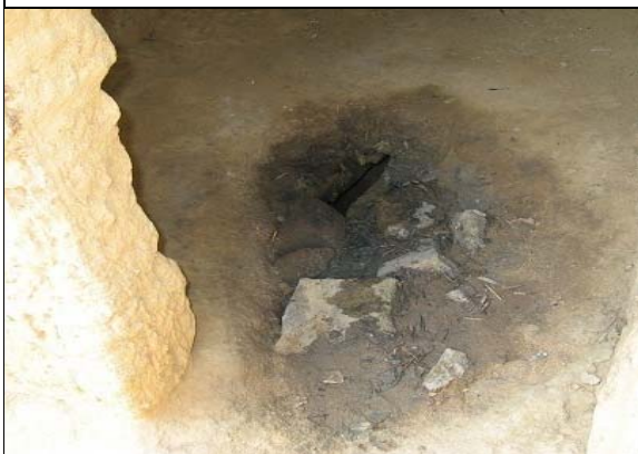
Pit latrine without slab (not washable)
