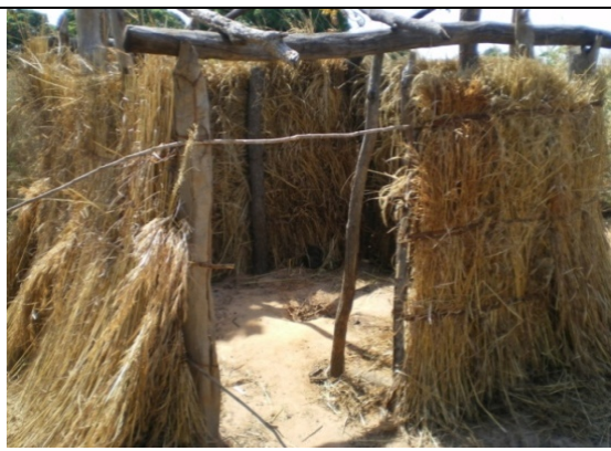
Pit latrine with slab (not washable)
