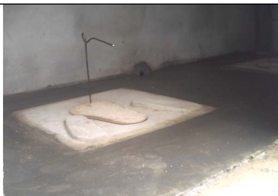
Pit latrine with slab (washable)
