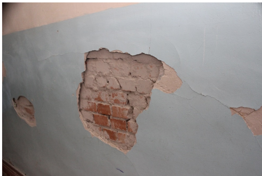
Figure IV.1. Illustration of damage in classroom walls
