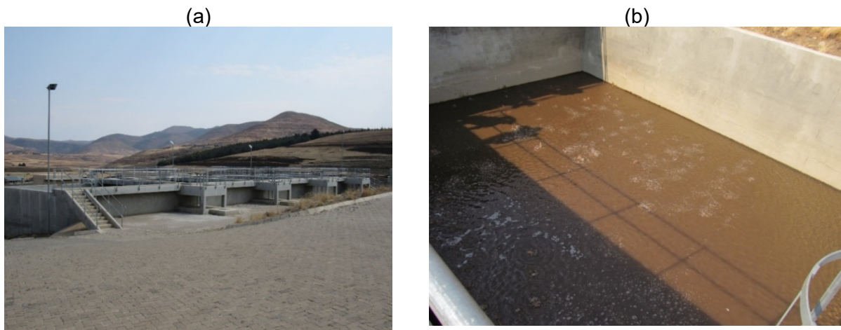
Figure 8. (a) Semonkong main sand filter beds; (b) Demonstration of uneven backwash
