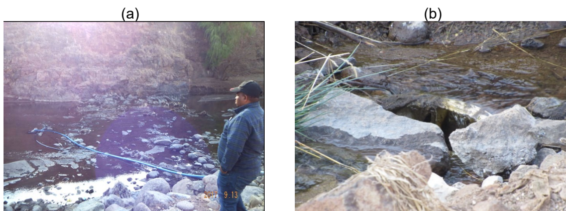
Figure 12. Mokhotlong (a) river abstraction by submersible pump; (b) spring intake cut open by WASCO
