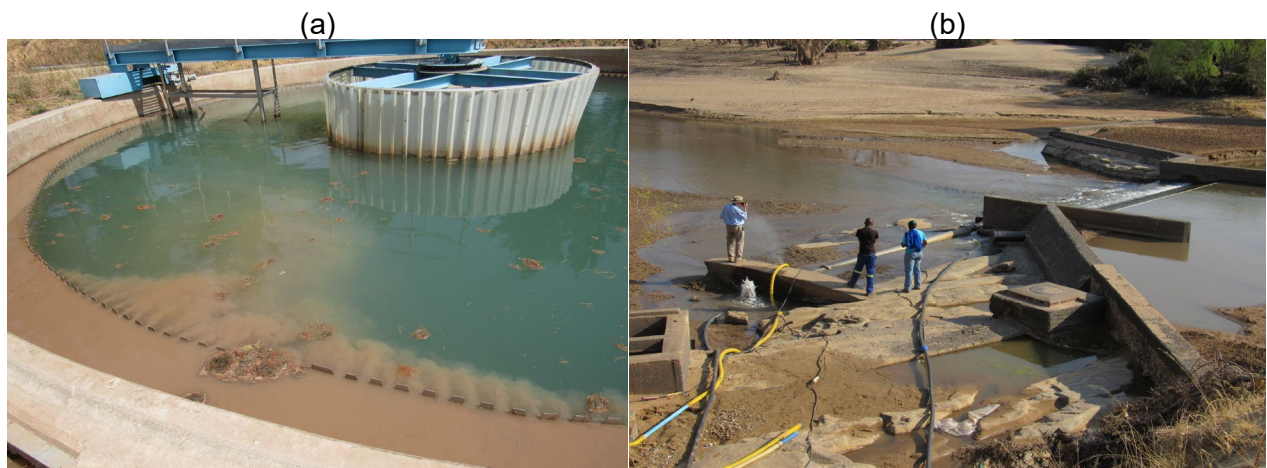
Figure 10. (a) Mafeteng Clariflocculator with excess sludge; (b) Mohale's Hoek improvised intake
