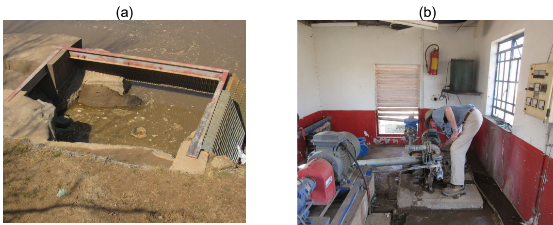
Figure 12. Mokhotlong (a) river abstraction by submersible pump; (b) spring intake cut open by WASCO
